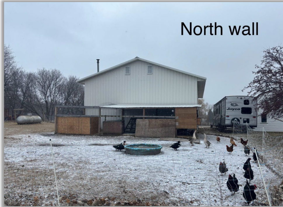
Figure 4 Photo of Existing Structure - North Wall
