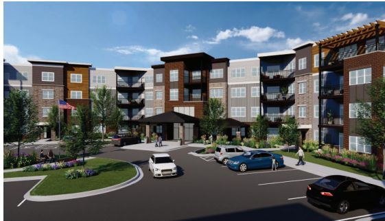
Class I materials: Multifamily Apartment
