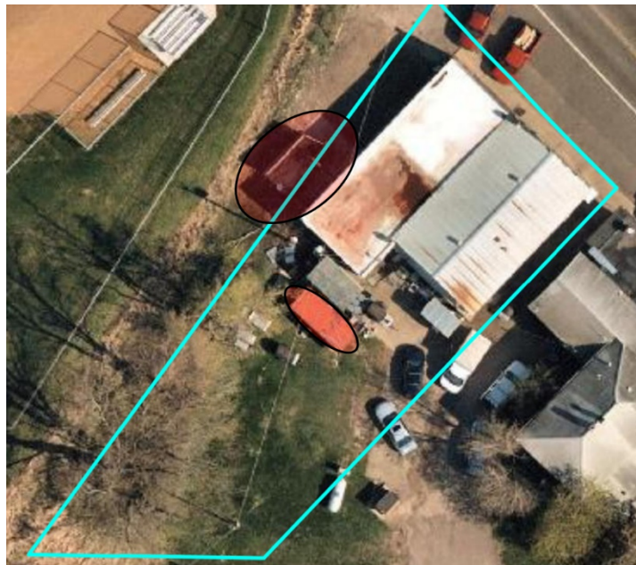
Figure 2 Image Showing Illegal Nonconformities
