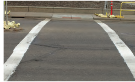
STANDARD/TRANSVERSE CROSSWALK PAVEMENT MARKINGS
