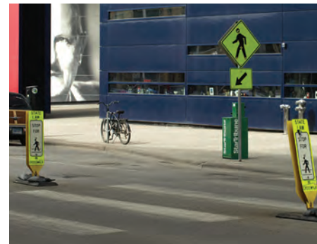
PEDESTRIAN CROSSING WARNING SIGN PLUS IN-ROAD SIGNS
