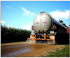
scatters the coarser aggregate, causing potholes, ruts, washboards, loss of profile, loss of ditch lines, and other problems. Wetting the road surface helps to keep dust-related problems in check. Moisture helps particles adhere to each other and to aggregates, allowing for optimum compaction. The trick is to keep the road moist.
